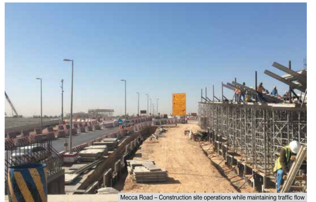
Mecca Road – Construction site operations while maintaining traffic flow
