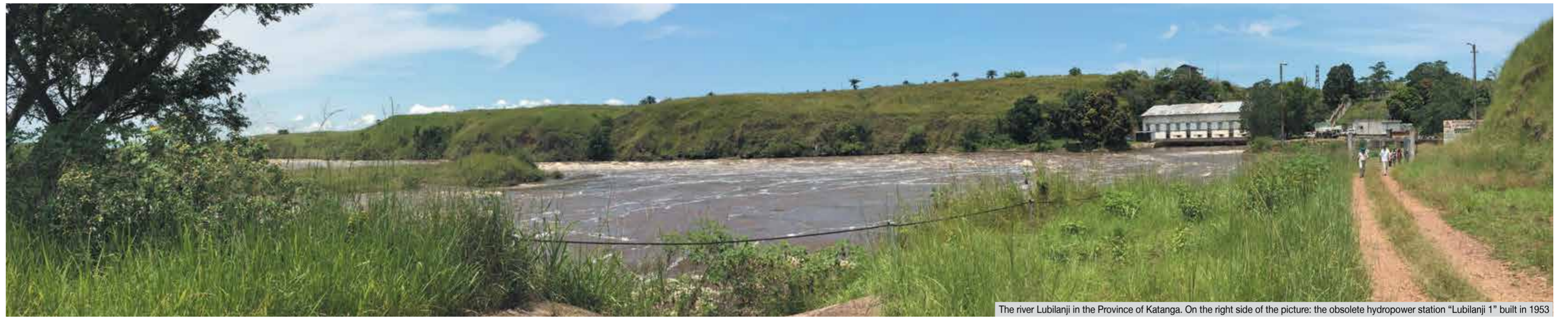
The river Lubilanj in the Province of Katanga. On the right side of the picture: the obsolete hydropower station "Lubilanj 1" built in 1953
